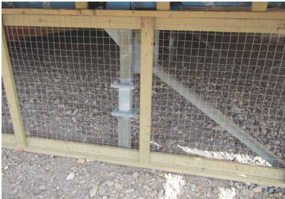
Figure 2.7.2.2 Extension added to piers on the community centre/daycare
