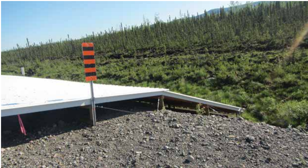
Figure 5.1 Snow shed used to preserve permafrost along the Alaska Highway
