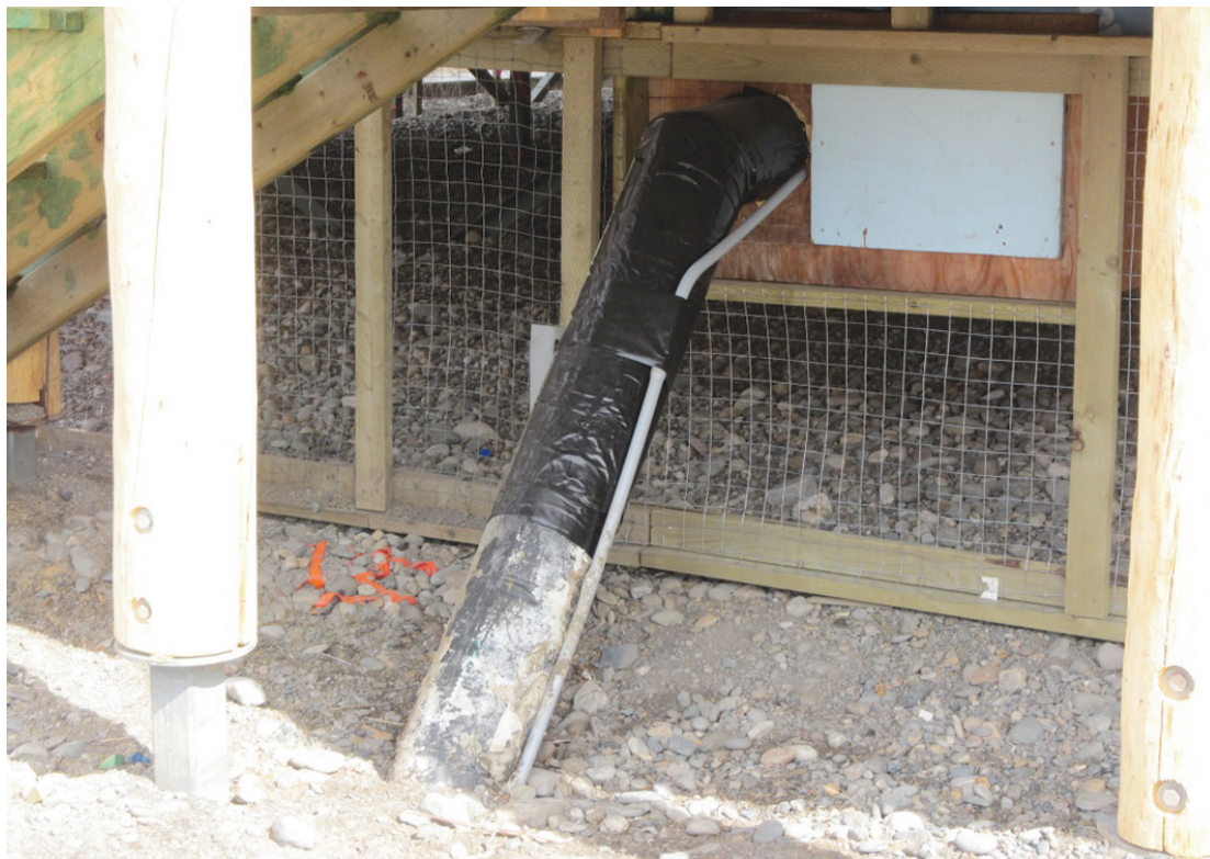
Figure 2.7.2.1 Repaired sewer line; sewer line had leaked for an unknown amount of time
