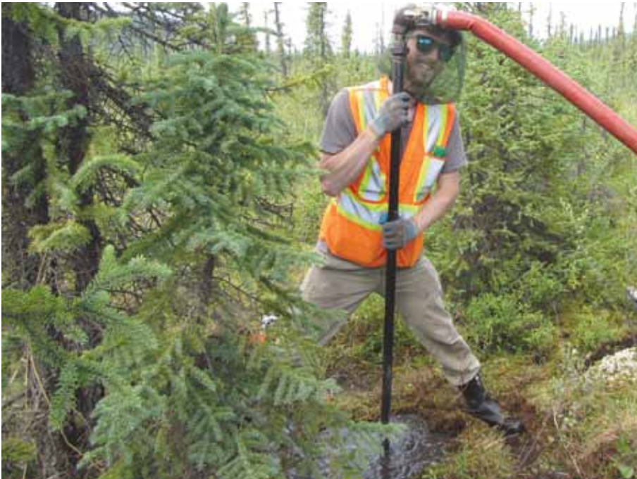
Water jet drilling at BH13, km 1896.3
