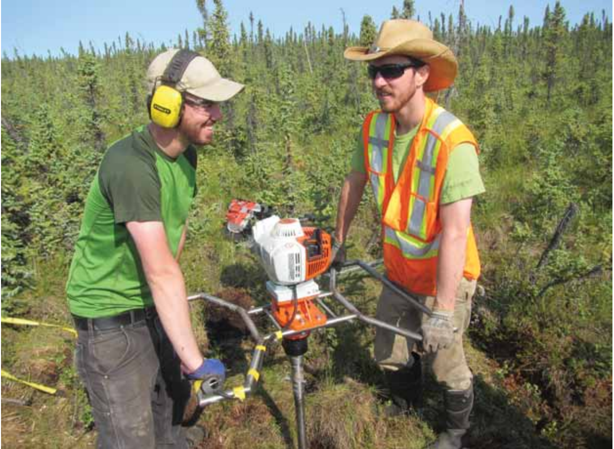
Drilling operation at BH20, km 1866.
