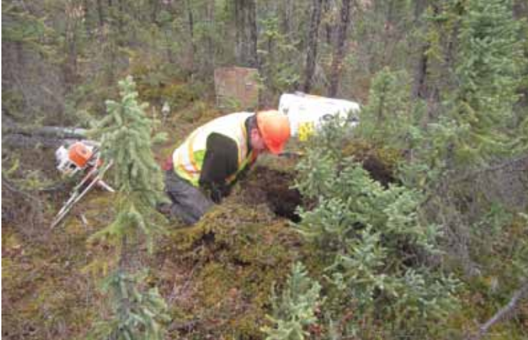
Drilling operation at BH05, km 1793.5.
