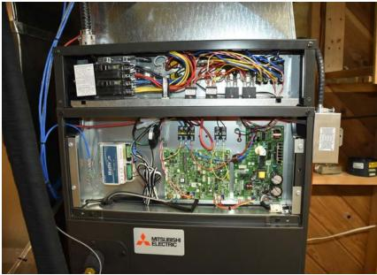
Figure 1: Inside of the indoor CCHP unit and the backup auxiliary heat with the power monitoring.
