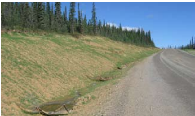
(i) Instead of track-walking and conventional seeding, this slope was hydroseeded (same slope depicted in photo d). Note how seeding was correctly extended all the way to the edge of the roadbed ( i.e. , seeded on both sides of the ditch). This will help stabilize the roadbed and prevent the spread of invasive plants. Also note the installation of temporary check dams in the ditch to slow the velocity of flowing water until vegetation is established.
