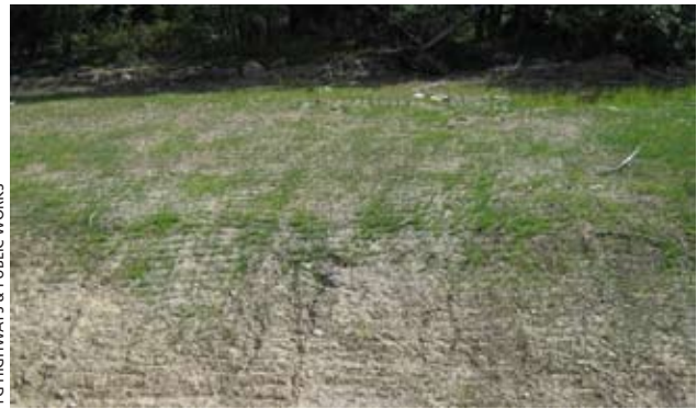
(h) This slope was successfully track-walked and seeded. A few rills formed but erosion was effectively halted as the grass became established.
