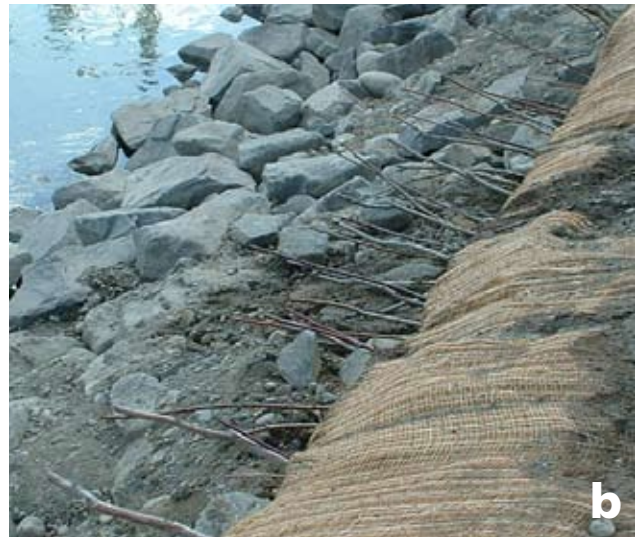
FIG 4.30 A three-pronged approach to bank revegetation. A willow hedge was constructed closest to the water's edge using stakes and an erosion control blanket (closeup in b), followed by mulch and seeding above. The willow bushes above the mulch were translocated from a donor site just a short distance away.
