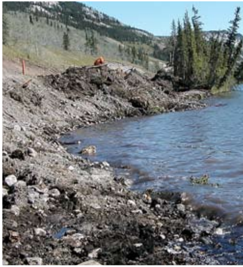
FIG 3.12a This stretch of lake shore was unintentionally disturbed during a road widening project. Without immediate erosion control and/or revegetation efforts, this roadbed will be undercut by wave action.
