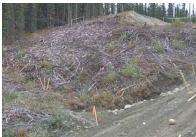
FIG 3.11 While this grubbed slope may look unkempt to some, the debris could be left in-place as an effective measure to protect against erosion. It also will keep the organic content of the site higher than if it is bladed and graded. Consequently, only a light seeding would be needed, and probably no fertilizer. If leaving large woody debris in place will present a hazard to future mowing and maintenance, it could be chipped and spread as a mulch on the site.
