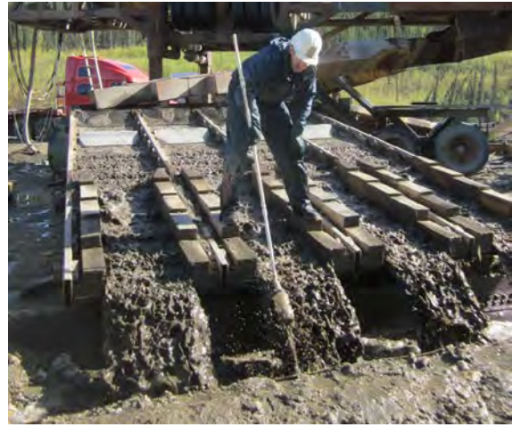
Figure 67 - Temporary Refit of Sluice.
