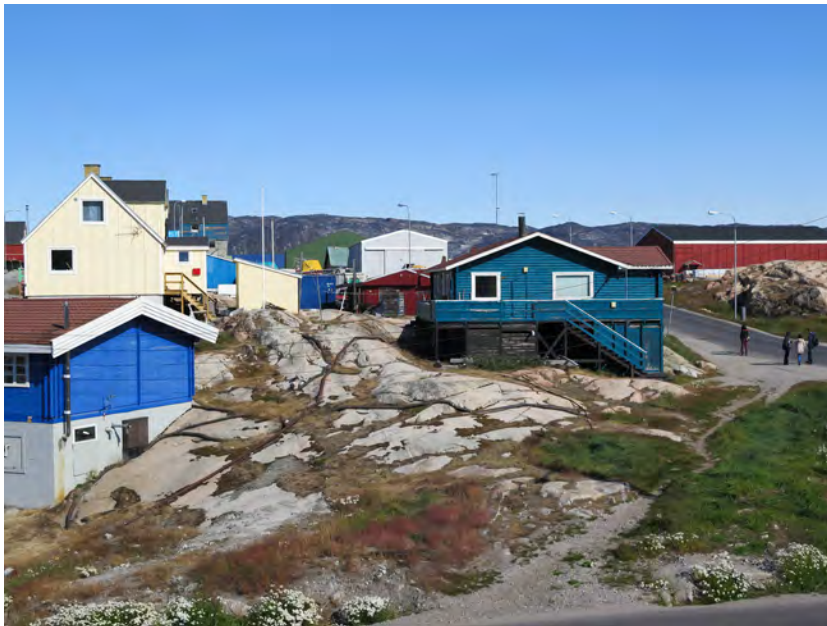
Figure C1. Houses in Ilulissat, western Greenland, built directly on bedrock.
