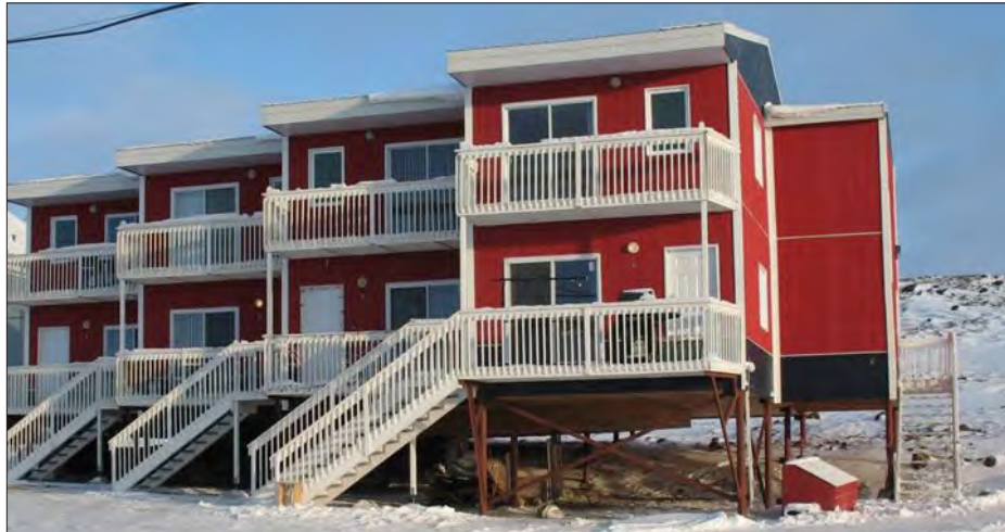
Figure C14. Example a steel-pile foundation in Nunavik (Gravel, 2012).
