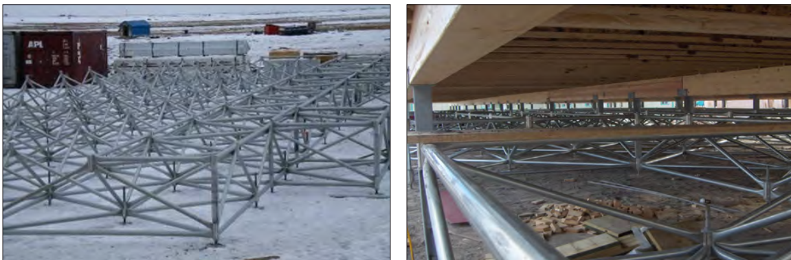
Figure C13. Examples of space-frame foundations in Nunavut (Barriault, 2012).
