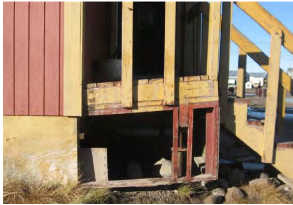
Figure F15. Examples of pile jacking in Nunavut (Barriault, 2012).
