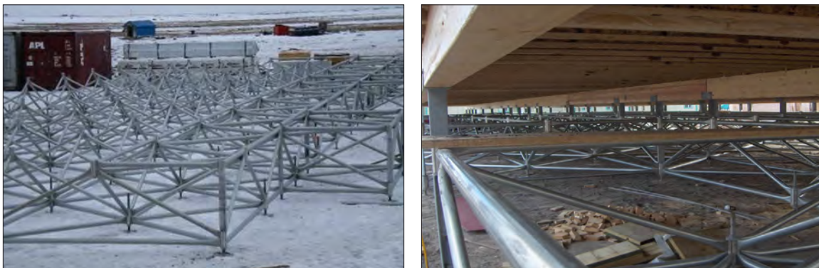
Figure F13. Examples of space-frame foundations in Nunavut (Barriault, 2012).
