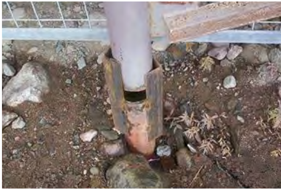
Figure F15. Examples of pile jacking in Nunavut (Barriault, 2012).
