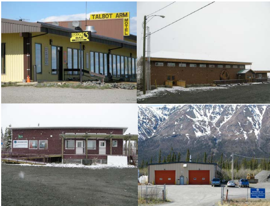
Clockwise from upper left: Talbot Arm Motel, Destruction Bay; Jacquot Hall, Burwash Landing; Sedata Business Centre, Burwash Landing; YG Maintenance Compound, Destruction Bay. Photos by Lisa Christensen.
